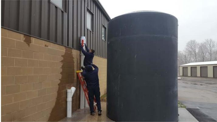
Public Works staff installs a pipe system to redirect rain water from the roof into a 5,000 gallon rain barrel.
